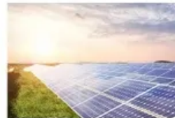
Energy Storage System
